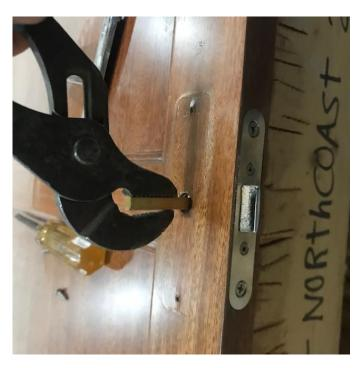
STEP 3: Pull the pin out and reinsert so that only a ¼" of the pin Gets reinserted and turn using the plyers in any Direction and open the door. When completed reinstall all items back together.
