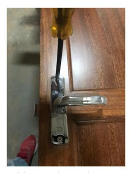
STEP 1: Use a Philip screw driver and remove top and bottom self tapping screws.
